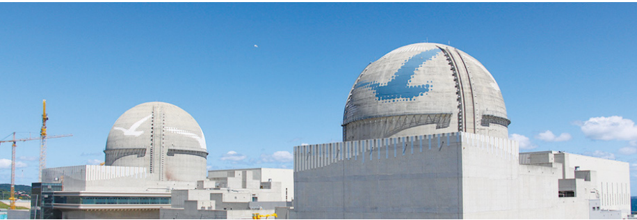
Nuclear Powe Plant
