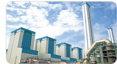
• Dangjin #1~4- World Best Project Awarded <US, Power Engineering, 2001>
